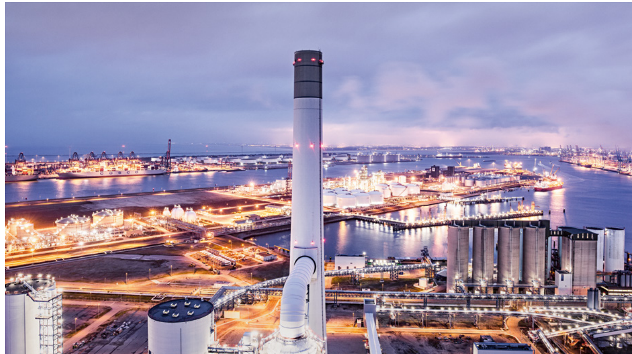
Maasvlakte Power Plant in the Netherlands.
