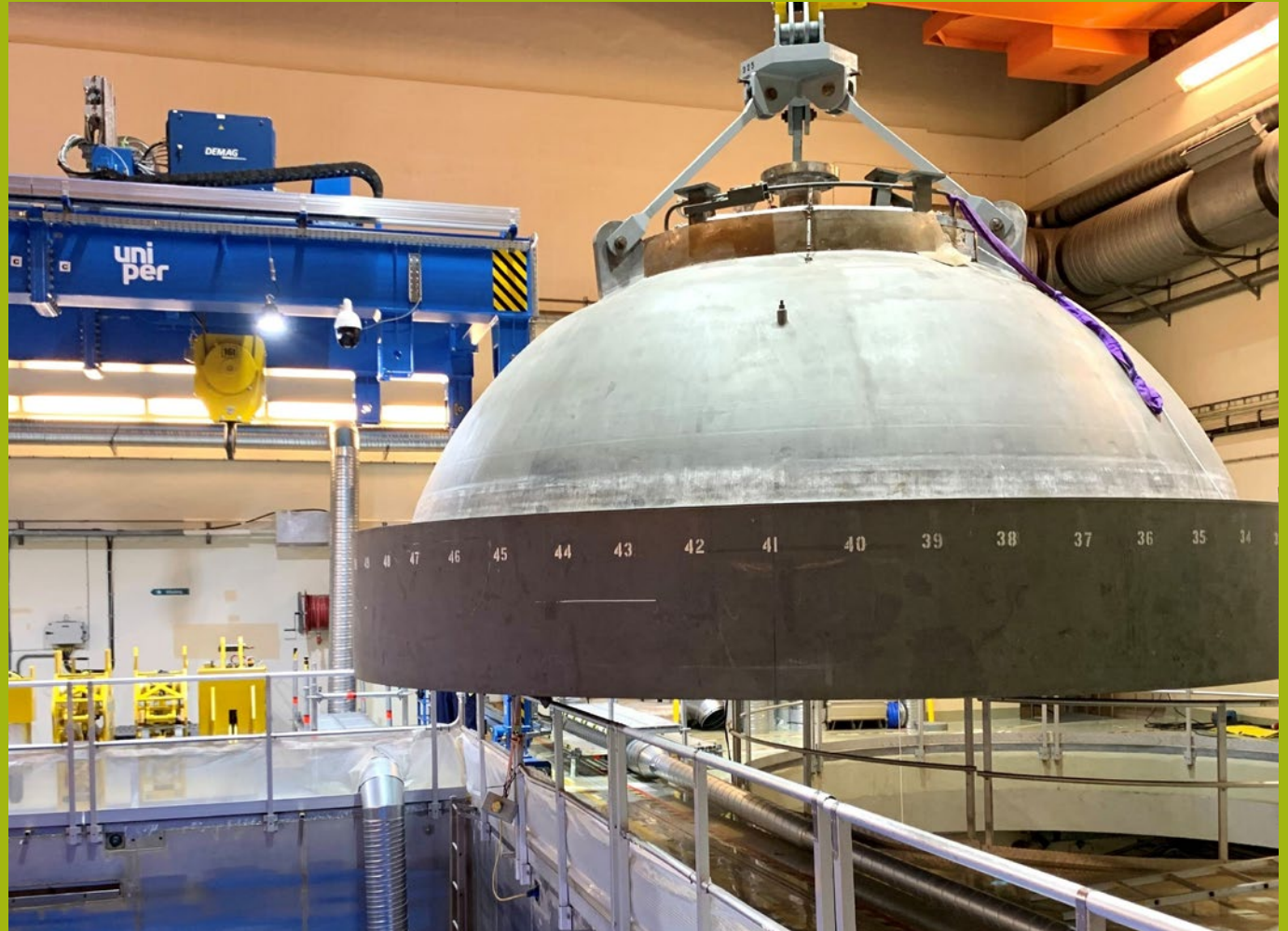
Lifting the reactor pressure vessel (RPV) lid.
