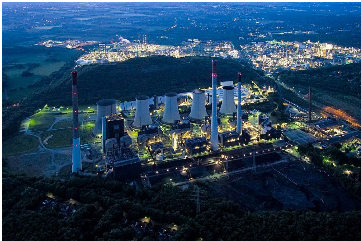
Scholven power plant, Germany.
